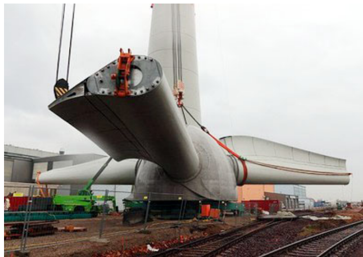
Figure 2-8: Rotor hub and blades [37]
