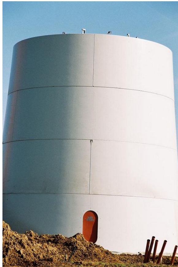
Figure 2-5: Enercon E-126 tower section [13]
